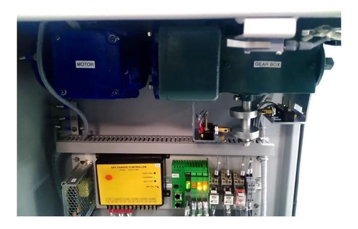
The Line Assist control cabinets are designed for remote control and local automation applications of switch disconnectors and other similar types with up/down operating movement. It can be combined with the advanced control modules for simple applications such as remote open/close operations and more sophisticated auto sectionalising schemes and measurements can be realised.
